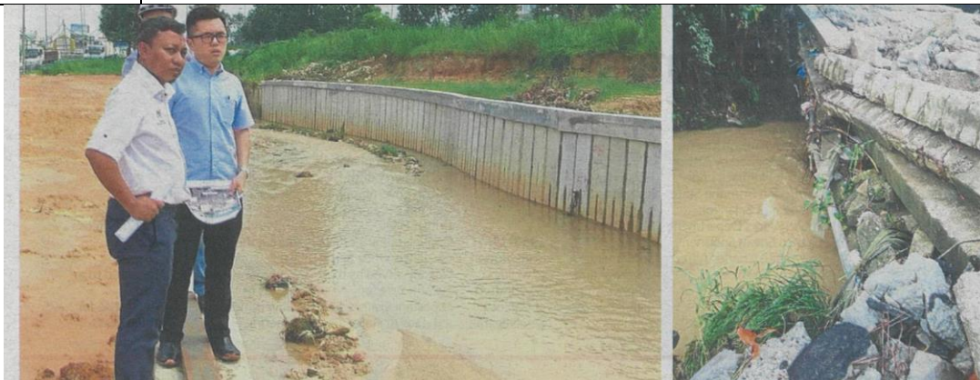
Chua (right) and Hasrul visiting the site of the river upgrading project.
